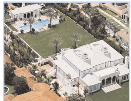
Construction completed, clearly dreams really do come true.
