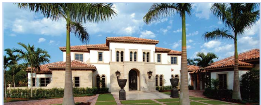
Keating-Moore Construction received the five PRISM Awards for Bella Vita (above), a French-Mediterranean home, completed in the gated Old Palm community in Palm Beach Gardens, Florida.
